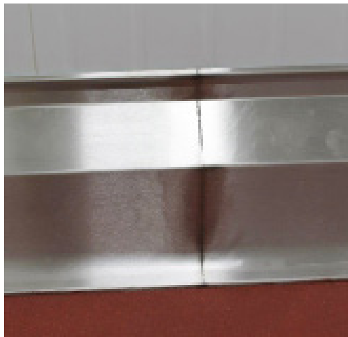
KE Wall Kerb Installation
