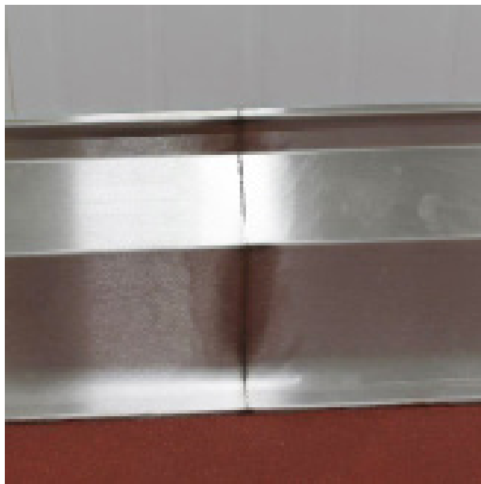
KE Wall Kerb Installation
